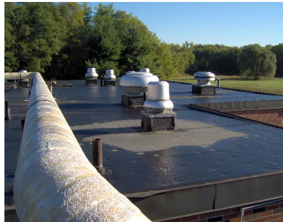
Main WWTB Building (not usable)
